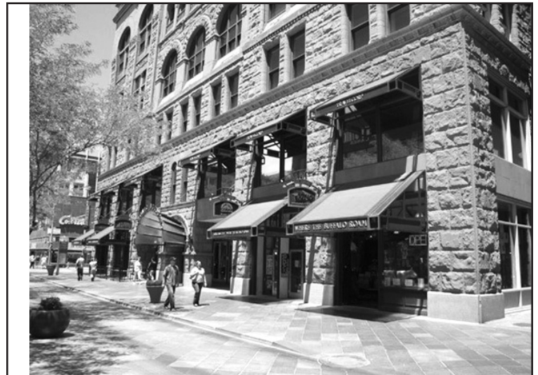
The Masonic Building's historic façade survived a 1983 fire that destroyed the rest of the structure.
